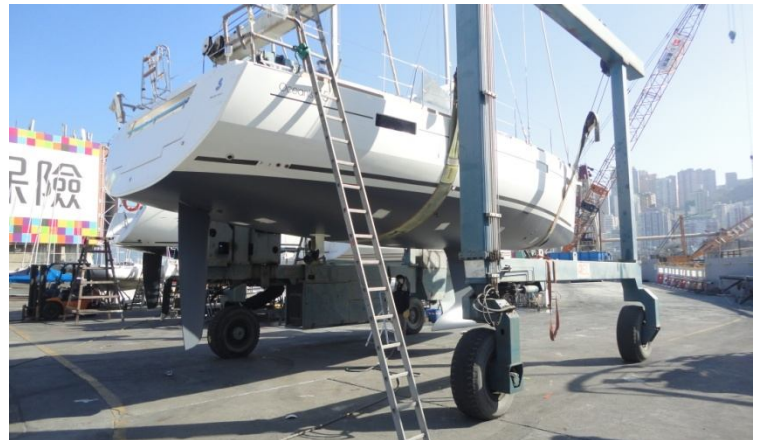
Boat held in slings for patches to be painted
